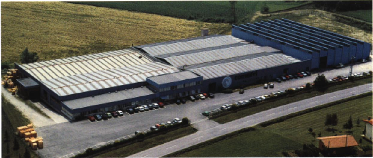
COMEFRI SpA's factory in Magnano in Riviera (UD), Italy with an 11.000 m 2 workshop where our radial fans for air-conditioning and general ventilation are manufactured.
